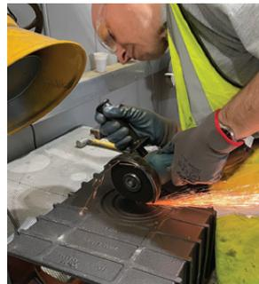
**3** Using an angle grinder with a 1mm disc attached, cut through the base of the channel separating it into four segments (see example above).
