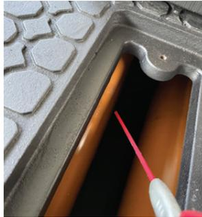
**2** Working on the right-hand access channel facing the road, take your lithium white grease can and spray the PVC pipes located in the access channel through the opening on top of the channel.
