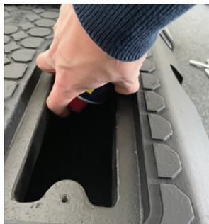
**2** Working on the right-hand access channel facing the road, take your lithium white grease can and spray down the expansion joint through the opening on top of the channel.
