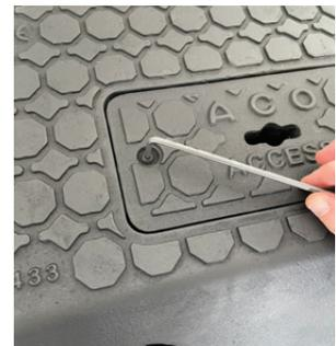
**4** Once you have lubricated both of the locations, the access cover should be placed back into position and fixed down.
